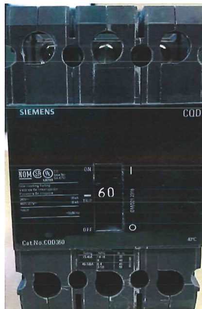
CQD breaker from 10/31/16 to 12/19/16 (Incorrect label)
